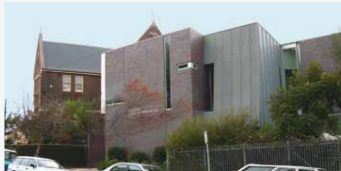
Flagstaff Crisis Accommodation Centre, Melbourne, VIC
