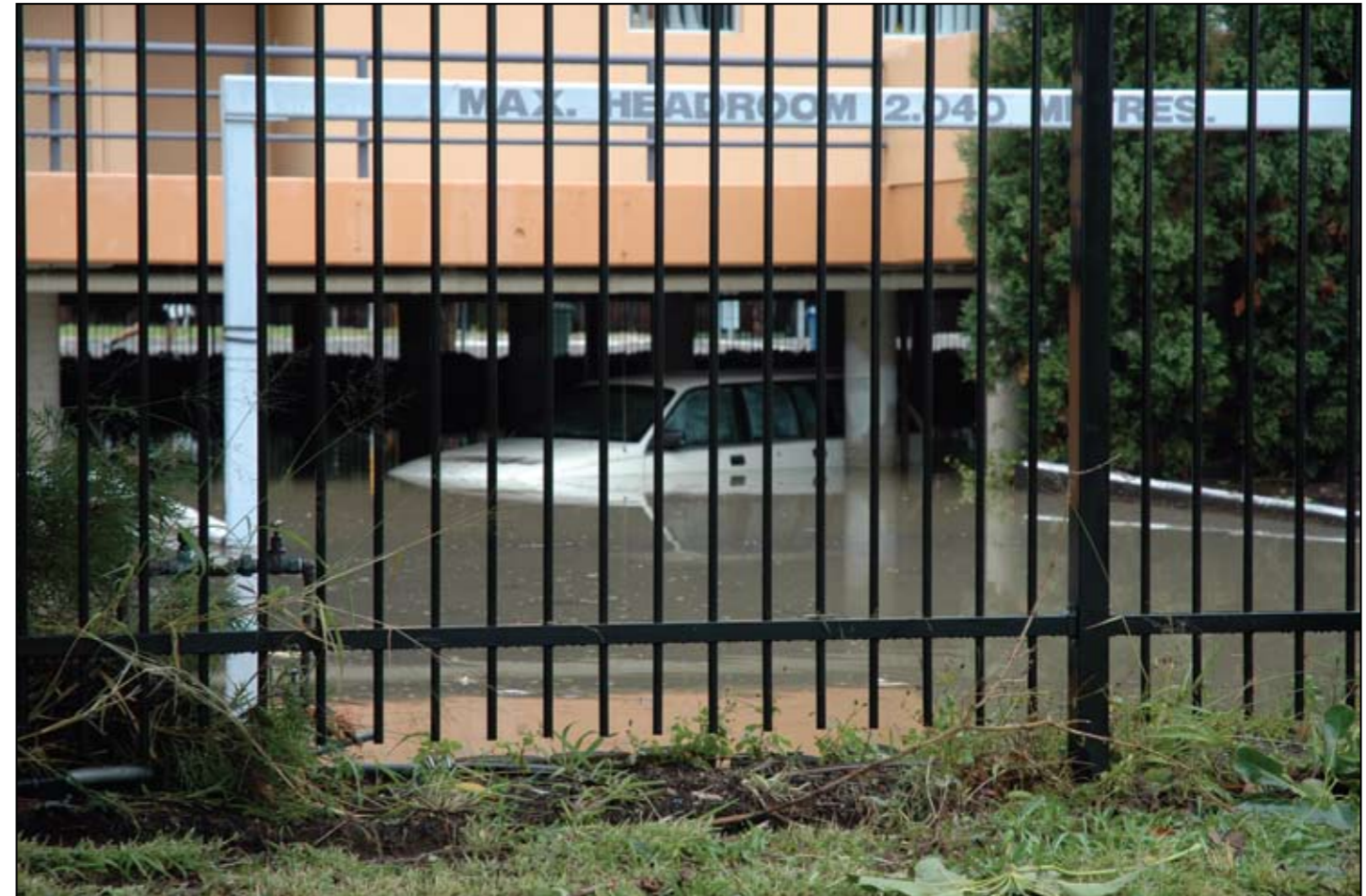
An underground car park in Newcastle resembles a swimming pool during the floods.
