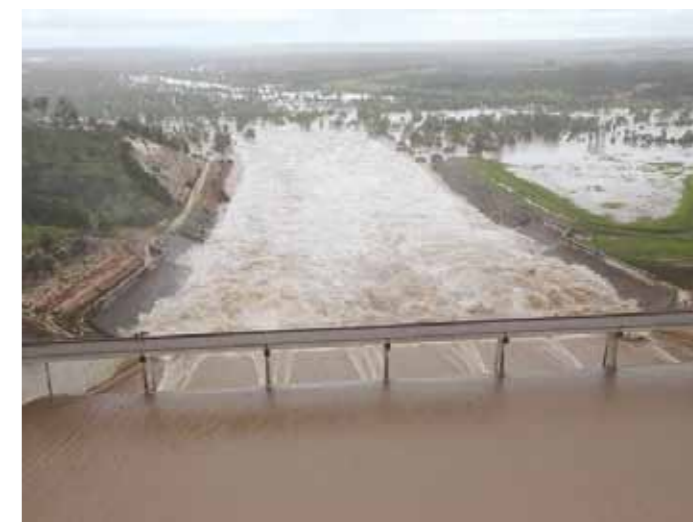
Fairburn Dam, near Emerald, overflowing above the spillway. At the height of the floods the dam was at 175 per cent capacity.
